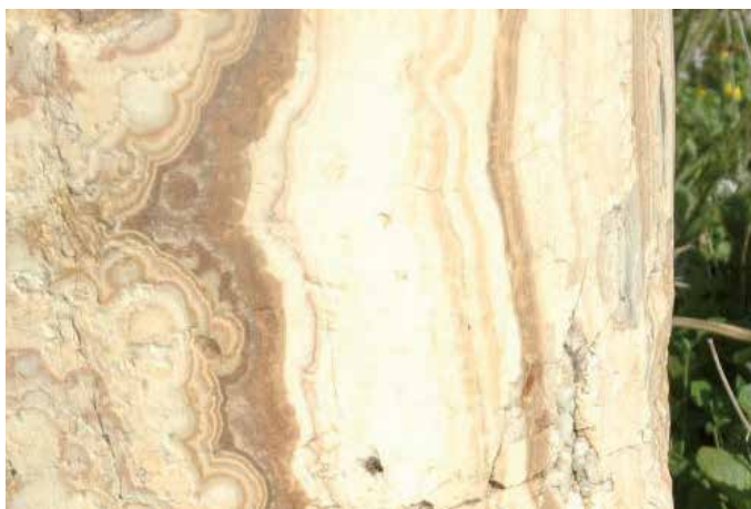
Fig. 2. Column drum of alabastro fiorito ; West Baths, Cherchel. Black surface staining partially removed.
